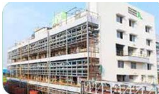
Agro &amp; Specialty Chemical Facility at Dahej-III
