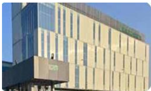
Pharma API Facility at Dahej-II (Gujarat)
